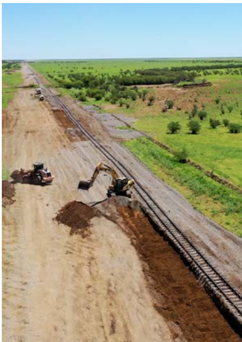
Image: Repair works to Mount Isa rail line.
