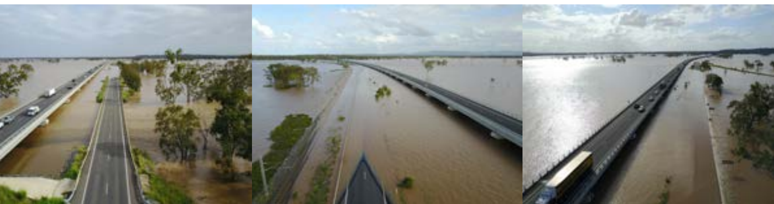
Images: 2017 Severe TC Debbie - Yeppen floodway.
